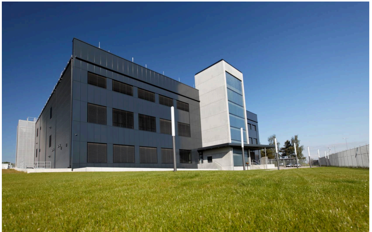
DATENCENTER Netcloud, Rümlang (Foto e-Shelter)
